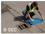
0 SEC Peel backing off underside of Plug Rug
