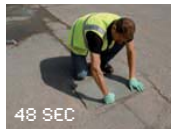
48 SEC Press edges down into surface
