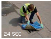
24 SEC Ensure Plug Rug overlaps drain
